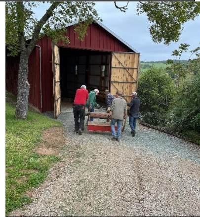
The hardworking removal and demolition crew move wagons into temporary storage.
