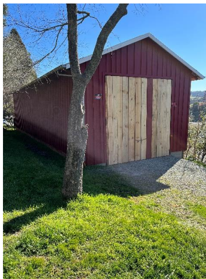
The Amador Historical Society storage building has doors. We're truly preserving the past and present for tomorrow.
